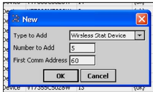
Figure 11: New Wireless TEC Device
